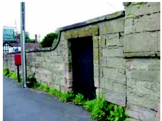
Wall to Tardebigge Court
