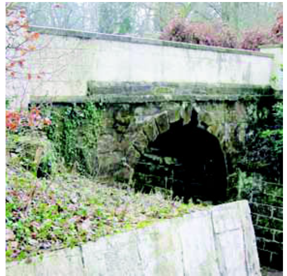
Sandstone bridge, Hewell Park
