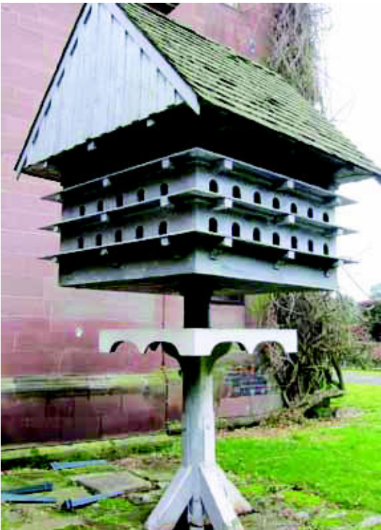
Dovecote to rear of Hewell Grange
